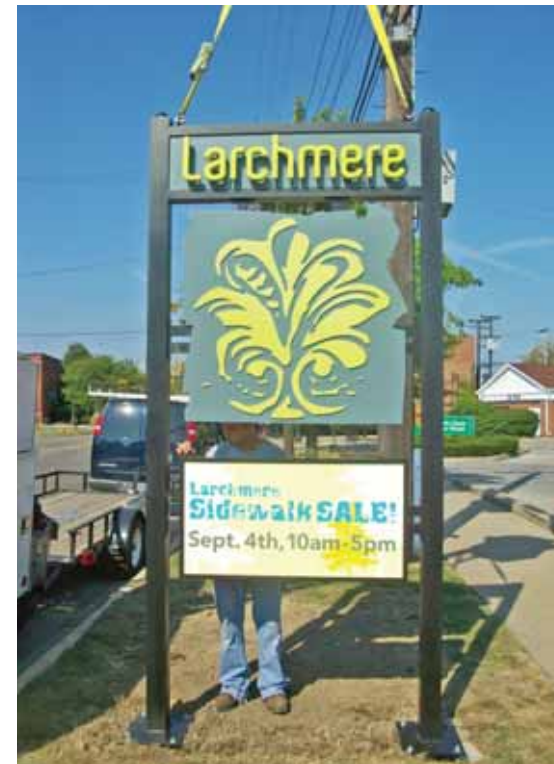
Installing one of the new Larchmere signs
