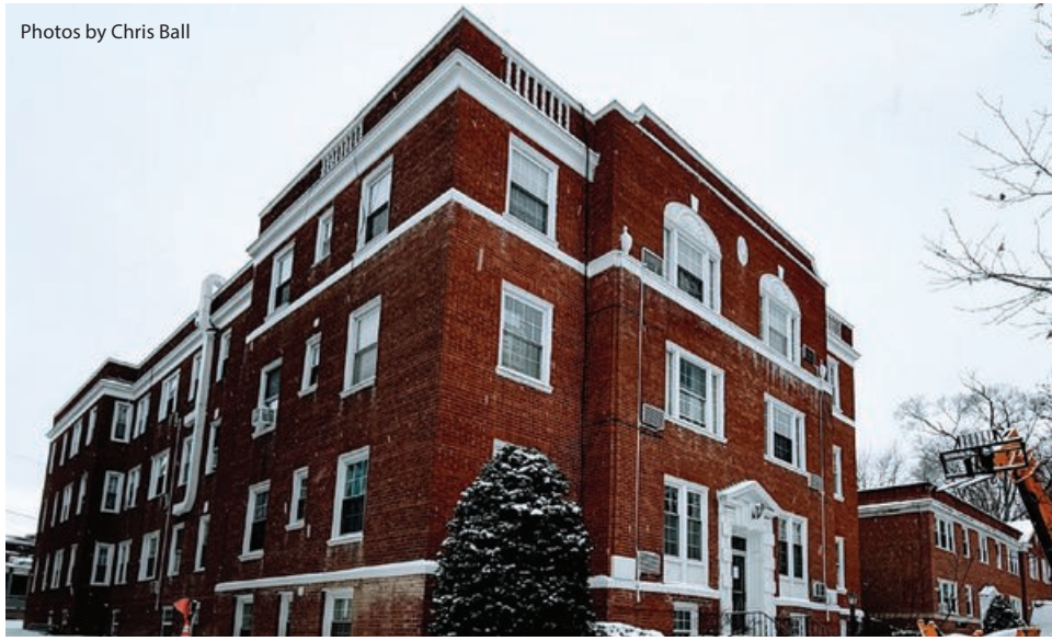
This apartment building at 13654 Fairhill Road was evacuated in early January first for no heat and then for no water.
